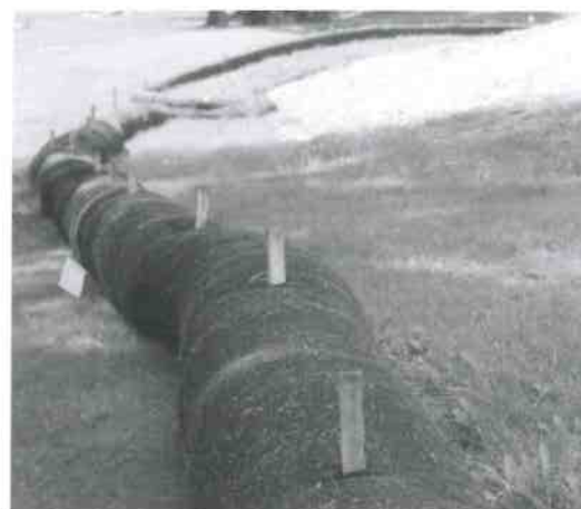
Compost filter sock
